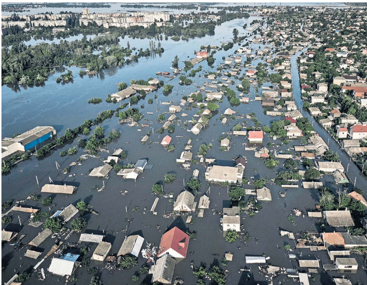
Deluge: streets stand flooded in Kherson on Wednesday after the Kakhovka dam wall broke
